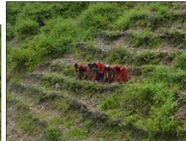
Brush layering is one technique preventing erosion and landslides
